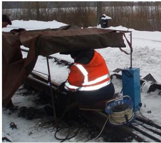
Fig. 5. Insufficient coverage of the welding area
